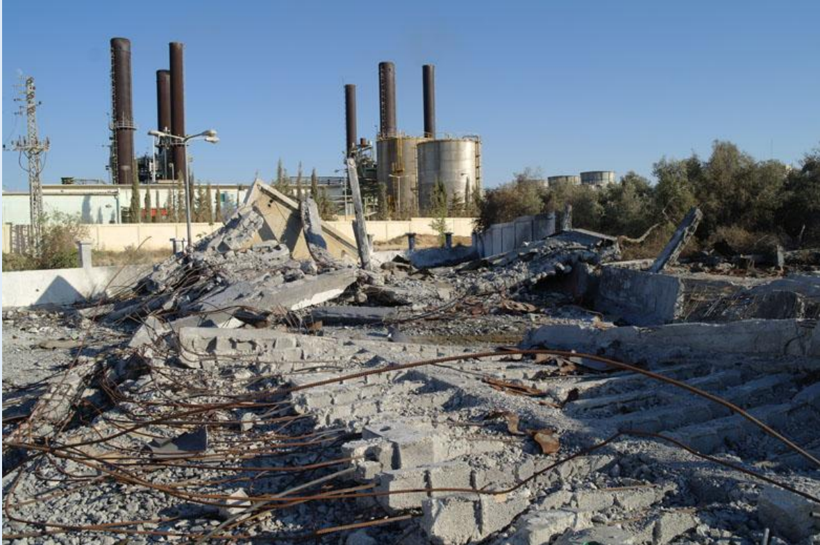
The damage caused by an Israeli attack on a pumping station in July 2011. In the background the only power station in Gaza, which was shelled in 2006 and again during the offensive of 2008-09 by the Israeli army.
